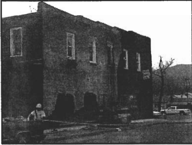
WALL SHOT "THE ORIGINAL WEST WALL OF THE 1860 BUILDING REVEALED TODAY."
