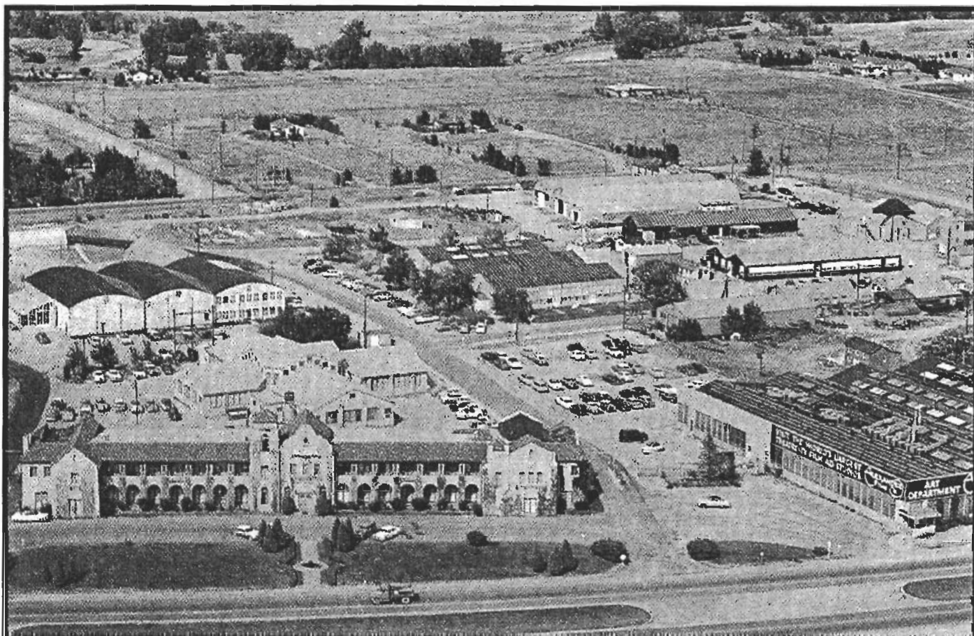
The Alexander Film Company at 3200 North Nevada Avenue. The four-winged building housed the Service Department managed by westsider Walter White
