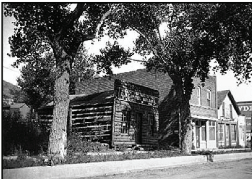
Courthouse #4 in Colorado City 1868
