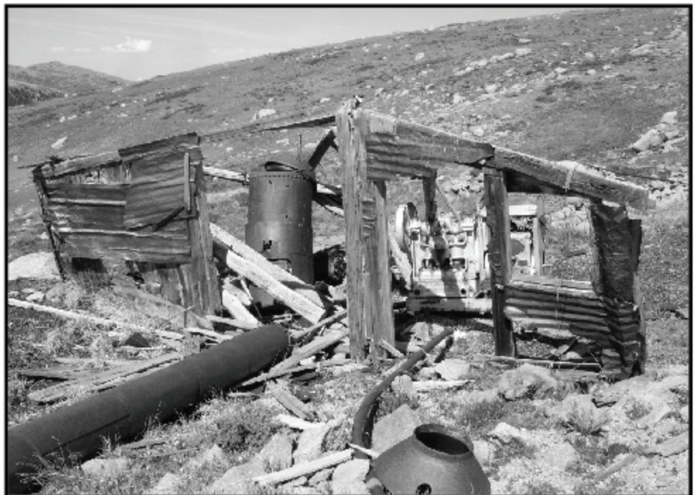
Pump house near Windy Point which housed steam and, later, gasoline powered pumps
