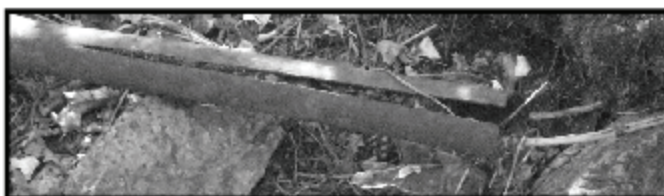
Cracked pipe from the Camp Vessey Water System.
